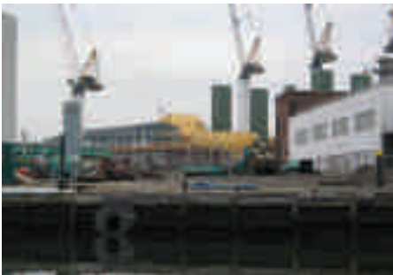
2003 Secondary Treatment Upgrade Construction at Newtown Creek WPCP Construction
