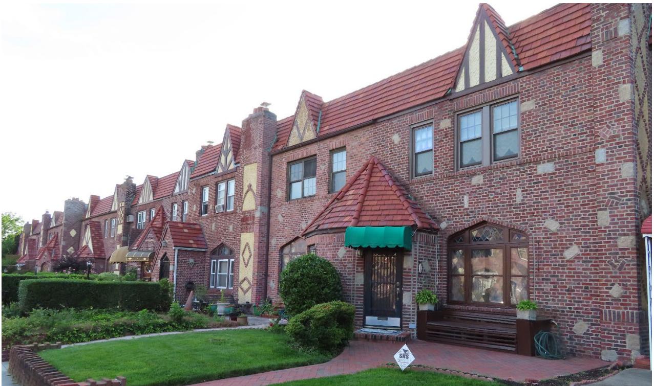
Figure 2: 222nd Street, east side Michael Caratzas, LPC, 2022
