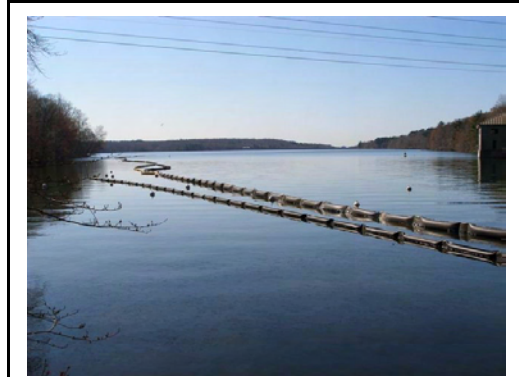
Figure 5.1 Catskill Upper Effluent Chamber turbidity curtain.
