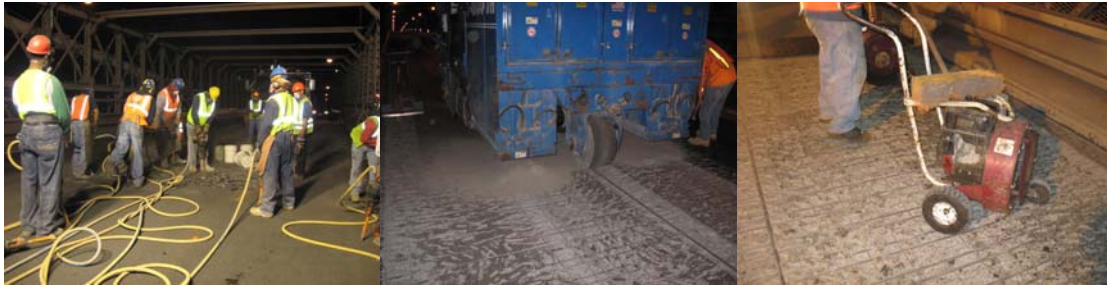
2008: Removing the Old Micro-Surfacing on the In-Bound Brooklyn Bridge. Shot Blasting for Surface Preparation. Cleaning the Roadway Surface. (Credit: Fouad Althaibani, Emad Shaker, and Sunil Desai)
