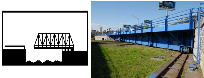
Borden Avenue Bridge. (Credit: Peter Basich).
