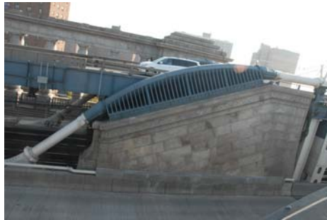
Manhattan Bridge Saddle. (Credit: Jagtar Khinda)
