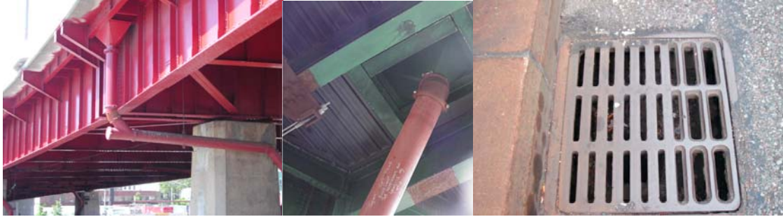
Scuppers on the Pulaski, Madison Avenue, and Brooklyn Bridges. (Credit: NYSDOT)
