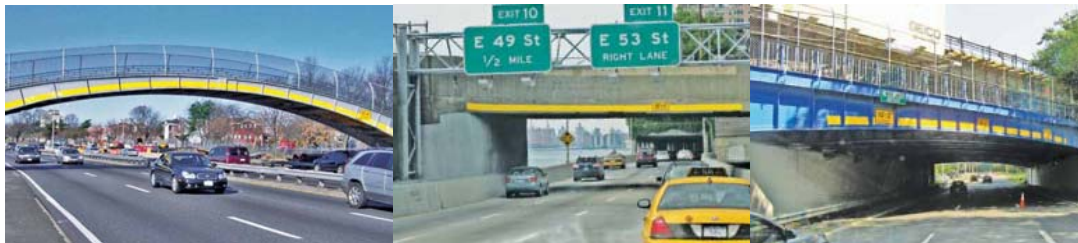
Retro-reflective Material Improves Visibility of These Low Vertical Clearance Bridges: 17 th Avenue Pedestrian Bridge Over Belt Parkway, East 60 th Street Bridge Over FDR Drive, and Westchester Avenue Bridge over Hutchinson River Parkway.
