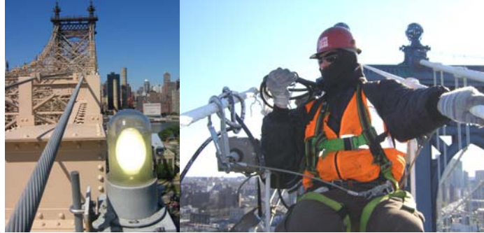
A Bulb of the Queensboro Bridge Necklace Lights. (Credit: Peter Basich) Repairing a Manhattan Bridge Necklace Light. (Credit: Hany Soliman)
