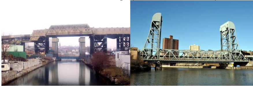
Ninth Street Bridge. (Credit: Bojidar Yanev) Broadway Bridge. (Credit: Bernard Ente)
