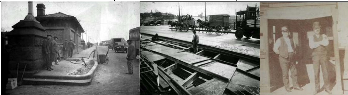
Willis Avenue Bridge Curbing and Road Repair in the Early 1920's. Gateman J. J. McDonough (on left), Great-Grandfather of Deputy Chief Engineer Russell Holcomb
