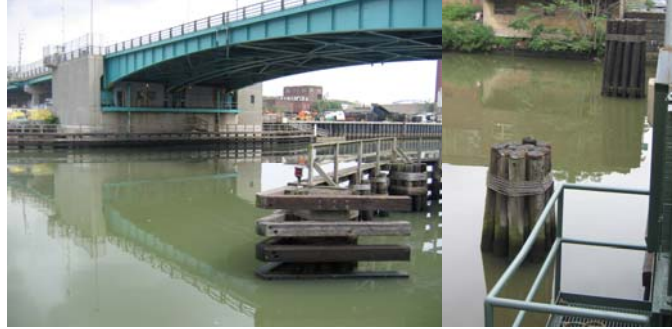
Greenpoint Avenue Dolphin & Fender System. (Credit: Peter Basich) Hunters Point Avenue Dolphins. (Credit: Michele N. Vulcan)
