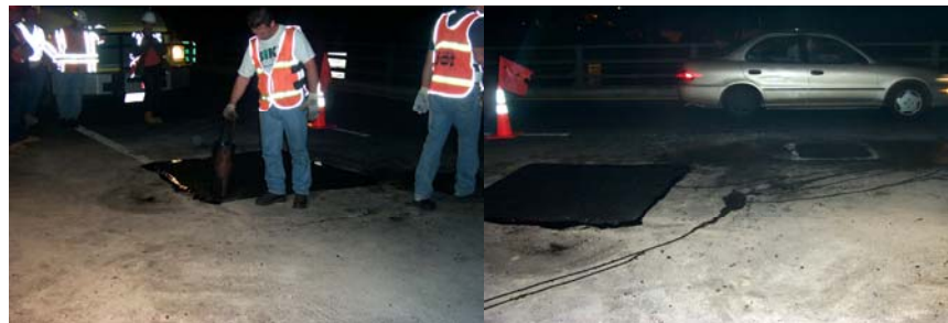
2005: Sealing the Edges of the Cutout With Asphalt Cement to Prevent Water From Seeping In. Closeup of Part of the Completed Concrete Deck Repair on the Eastbound BQE. (Credit: Anthony Napolitano)
