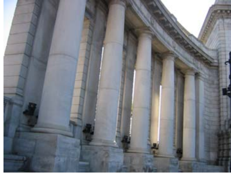
Manhattan Bridge Colonnade. (Credit: Peter Basich)
