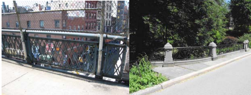
Manhattan Bridge Railing. (Credit: Russell Holcomb) Greywacke Arch Railing.
