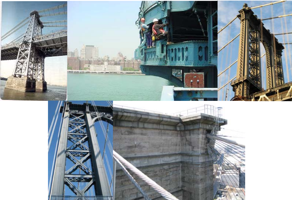
Williamsburg Bridge Tower. (Credit: Peter Basich) Inspectors on Manhattan Bridge Tower. (Inspector Credit: NYSDOT) Manhattan Bridge Tower. (Credit: Michele N. Vulcan) Manhattan Bridge Tower Detail. (Credit: Russell Holcomb) Brooklyn Bridge Brooklyn Side Tower Detail. (Credit: Jagtar Khinda)
