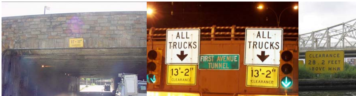
Woodhaven Boulevard Bridge Eastbound, United Nations – 1 st Avenue Tunnel, and Macombs Dam Bridge Vertical Clearance Postings. (Credit: NYSDOT)
