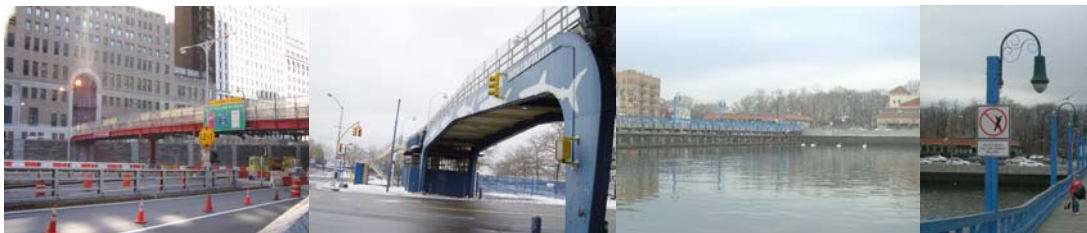
Morris Street, West 8 th Street, and Ocean Avenue Pedestrian Bridges.
