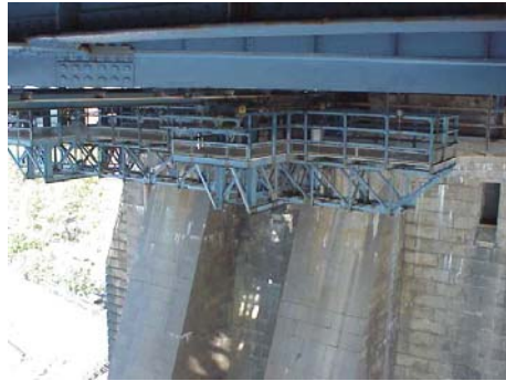
Manhattan Bridge Traveler. (Credit: NYSDOT)
