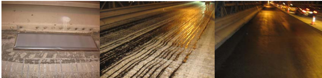
2008: Covering all the Drainage Systems Before Applying the Micro-Surfacing on the In-Bound Brooklyn Bridge. Applying the Tack Coat for the Micro-Surfacing. Applying the New Micro-Surfacing Materials. (Credit: Fouad Althaibani, Emad Shaker, and Sunil Desai)
