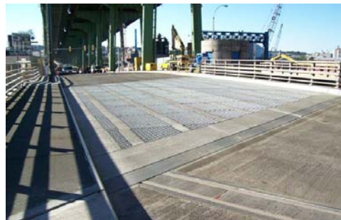
Hamilton Avenue Bridge Deck. (Credit: NYSDOT)
