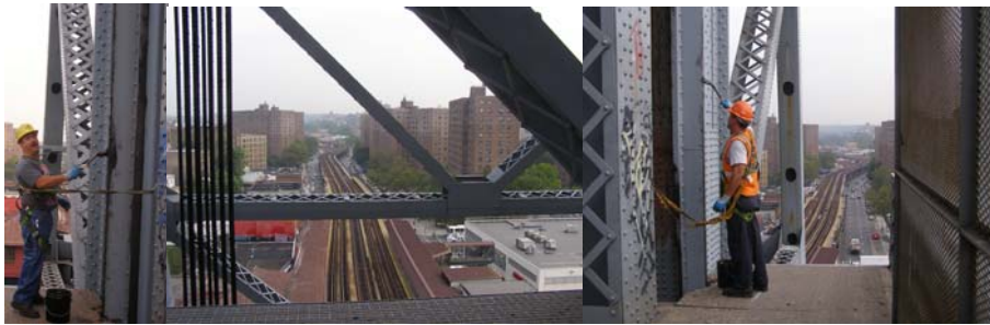
Cleaning and Lubricating the Broadway Bridge. (Credit: Reza Taheri)
