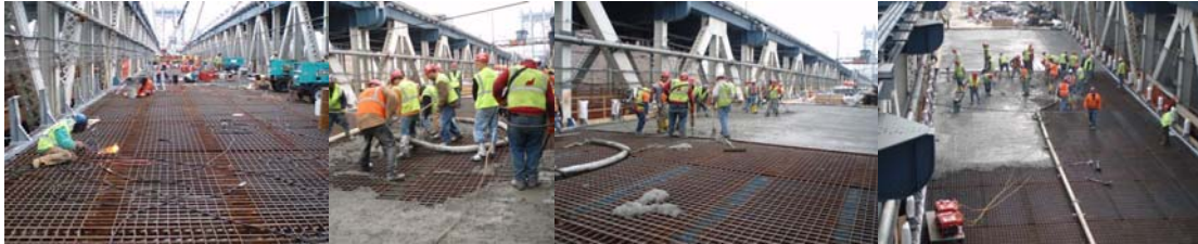
Installation of Full Width Grid Deck Panels on the Manhattan Bridge Lower Roadway in 2006. Pouring the Concrete.
