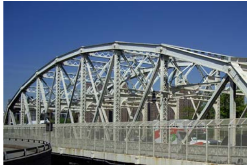
Macombs Dam Camelback Truss.
