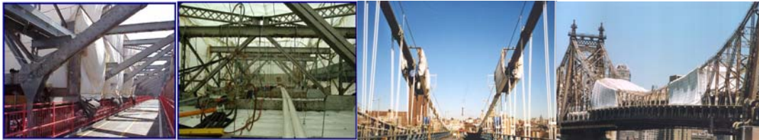
Containment Examples. Manhattan Bridge - Painting Containment Structures on the Cables of the Manhattan Approach Span. 2005: Queensboro Containment. (Queensboro Credit: Peter Basich)
