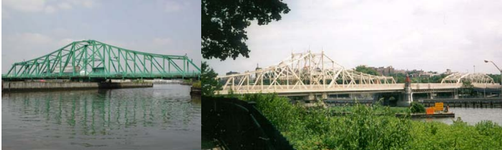
Grand Street Bridge. (Credit: NYSDOT) Macombs Dam Bridge. (Credit: Michele N. Vulcan)
