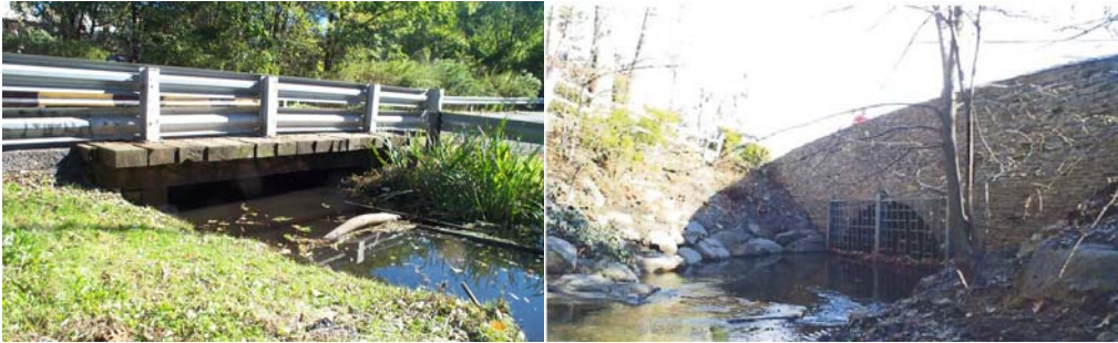
Idlease Place Culvert. Sweet Brook Road Culvert.
