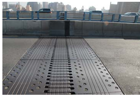
Manhattan Bridge Finger Dam. (Credit: Jagtar Khinda)
