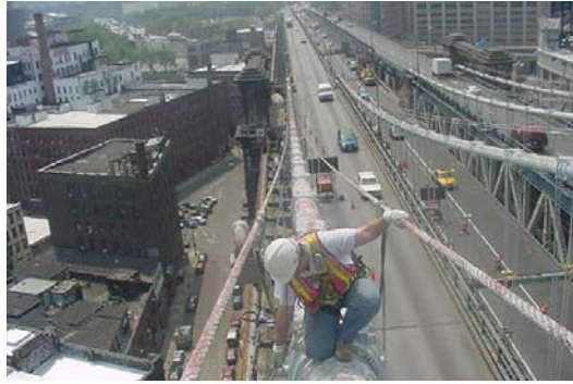
Inspector on Manhattan Bridge Cable. (Credit: NYSDOT)
