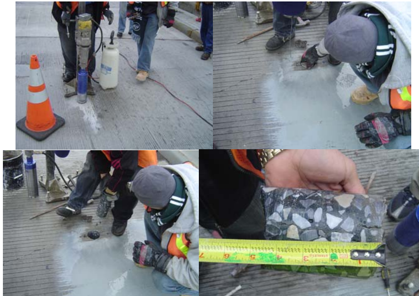
Removing a Core From 252 nd Street Bridge over Henry Hudson Parkway in January 2009. (Credit: Masroor Mahmood)
