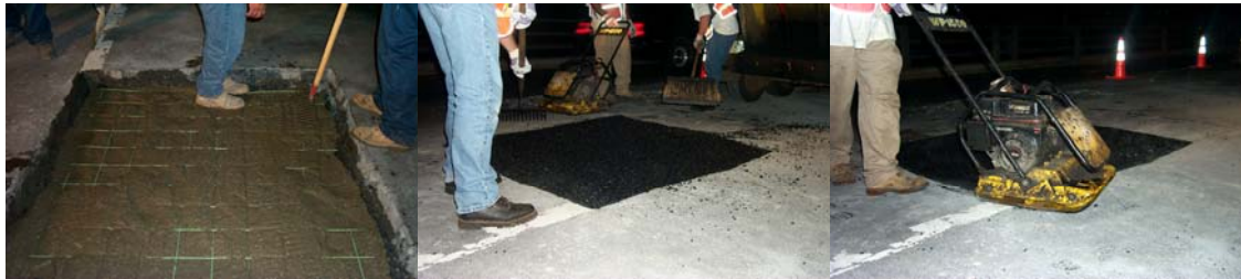
2005: Installing New Concrete With Rebar in the Cutout on the Eastbound BQE. Rolling and Tamping the Asphalt on the Eastbound BQE. (Credit: Anthony Napolitano)
