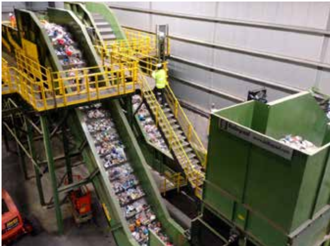
Sims Municipal Recycling processes NYC's residential and school recycling.
