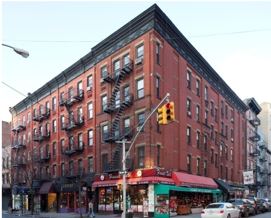
177 to 171 Bleecker Street Built in 1887-88 and designed by Alexander I. Finkle
