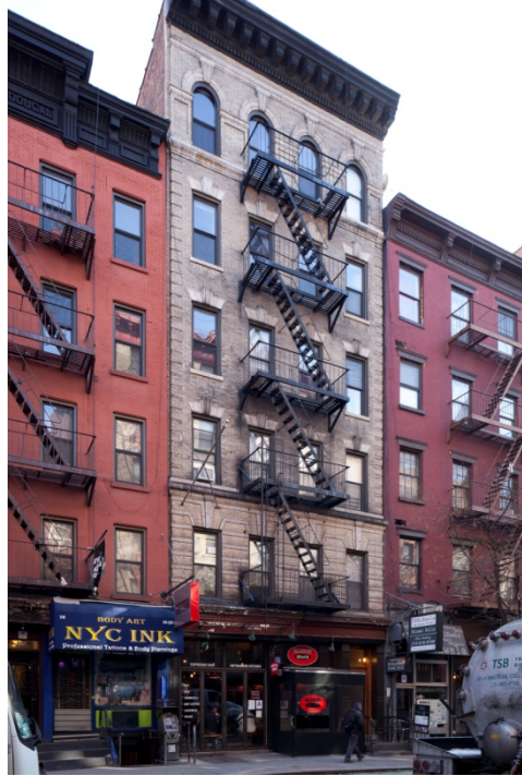
114 MacDougal Street Built in 1899-1900 and designed by John Philip Voelker
