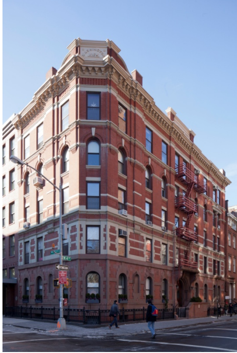
39½ Washington Square South Built in 1889-90 and designed by Thom & Wilson
