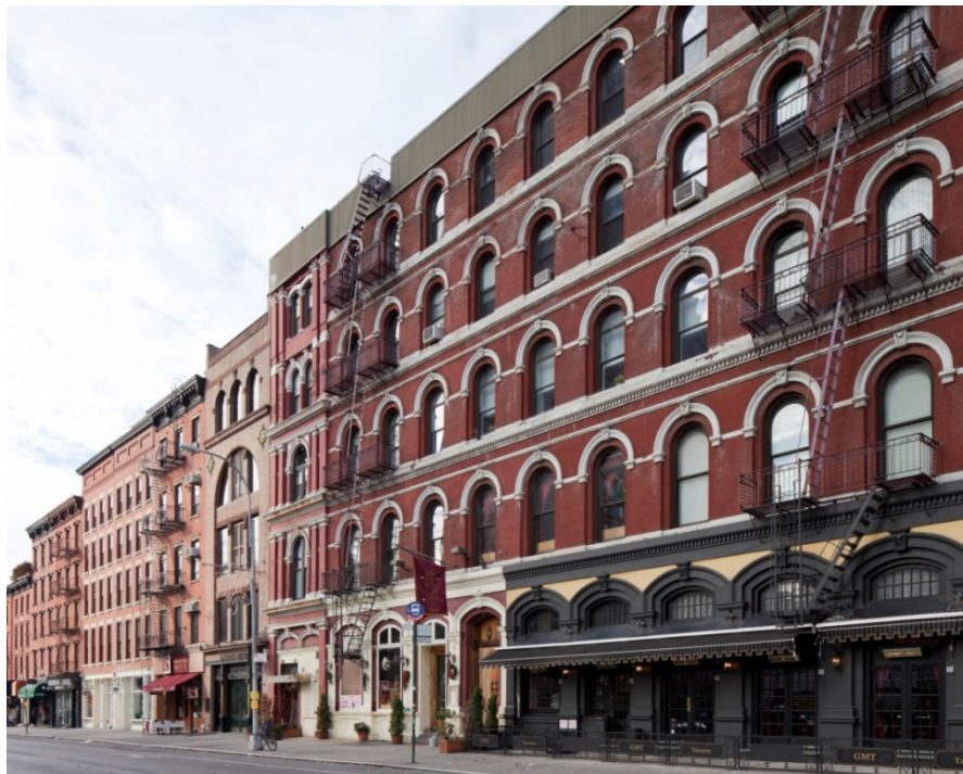
Streetscape along LaGuardia Place with 510 LaGuardia Place in foreground (1871-72, Henry Fernbach)
