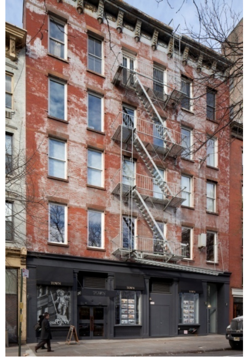
528 LaGuardia Place Built in 1884 by J. V. Close & Bro., builders
