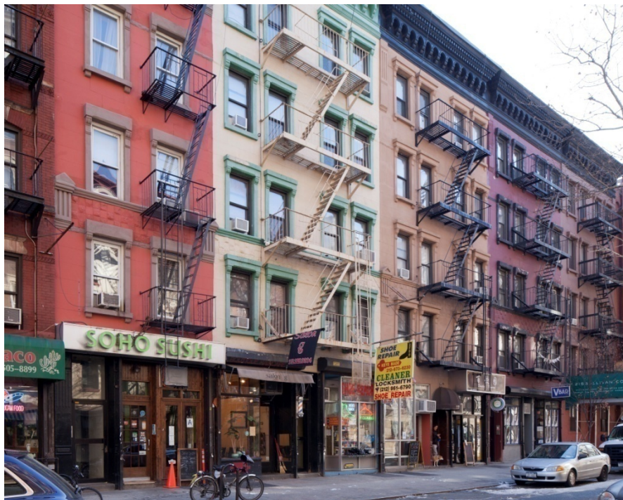
231 to 223 Sullivan Street Built in 1886-87 and designed by William B. Tuthill
